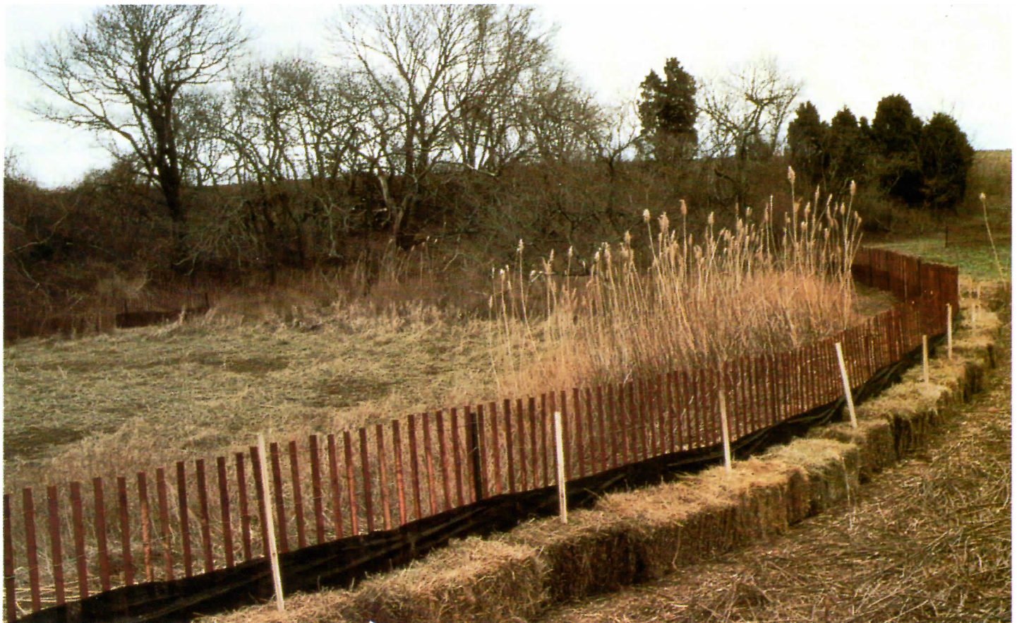
Erosion control methods employed around the wetlands.
